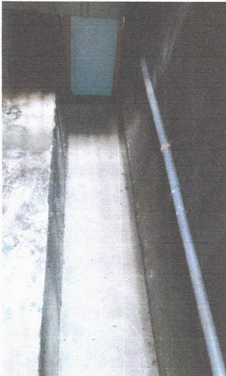
Drainage after covered
